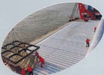
长江航道铺排工程 The Yangtze River waterway laying engineering.
